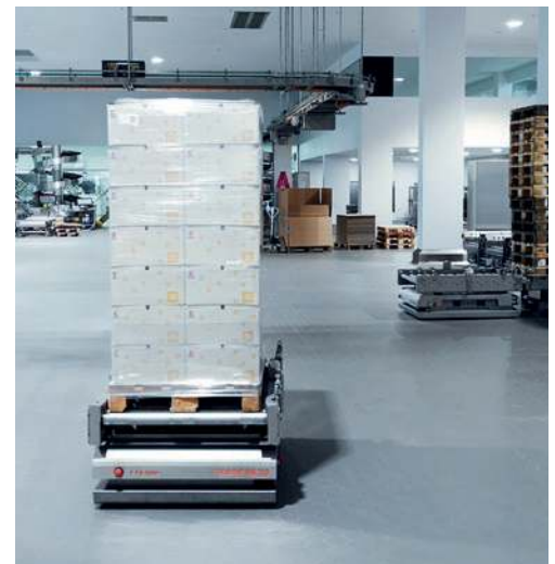
➤ The TRAPO Transport Shuttle as a link for storage and loading.
